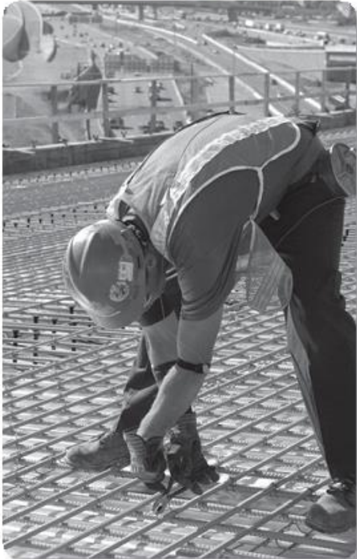
Problem: Tying rebar by hand
