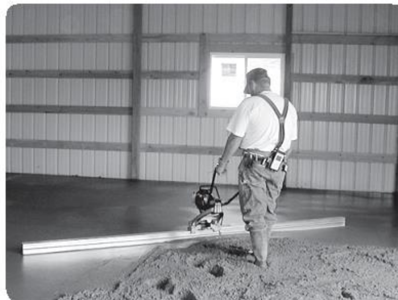
Solution: Motorized screeding
