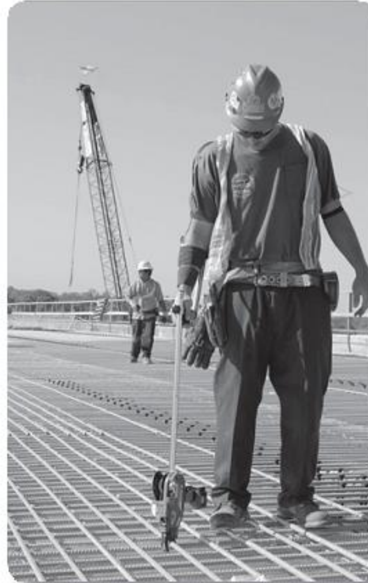
Solution: Rebar-tying tool with extension handle
