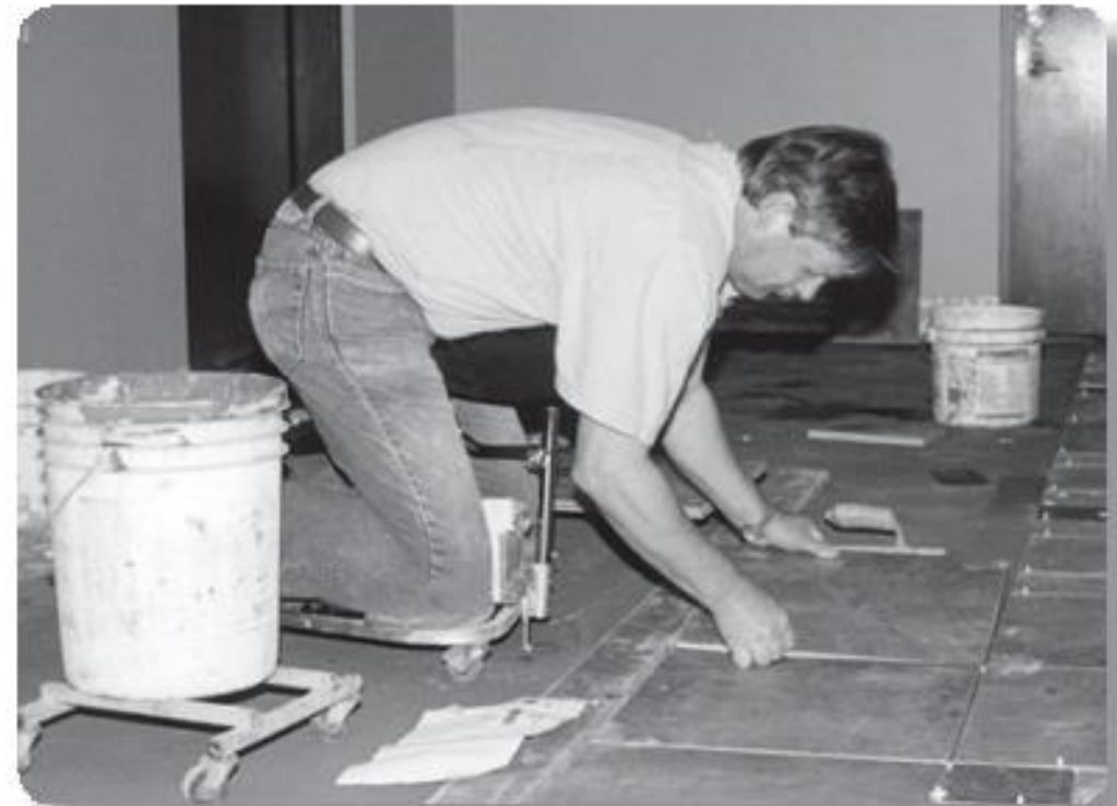
Solution: Laying tile with kneeling creeper
